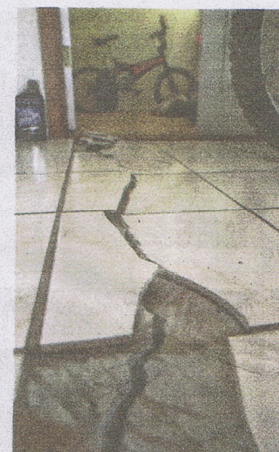
Expansive soil can lead to cracks in the foundation. THE REPUBLIC
